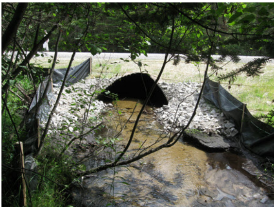
East Branch Tributary at Trask Lake Road improvements completed in 2015
