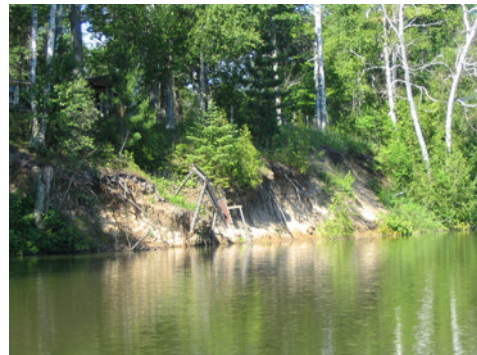
Erosion site on the Pine River in need of stabilization
