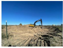
October 18, the excavation of soil was initiated at FT002, over 20,000 tons have been removed to date. PFAS contaminated soil is being removed down to the water table to reduce the amount of PFAS that can reach the water table and evenually reach Clark's Marsh. The excavtion will be refilled with uncontamnated soil. The contaminated soil is being taken to a special hazardous waste landfill downstate for disposal.
